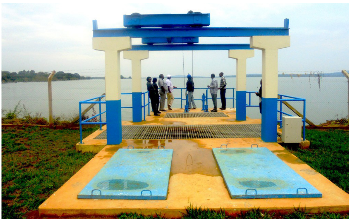
The water intake for Sengerema water treatment plant in Tanzania constructed under the LVWATSAN II Project.
