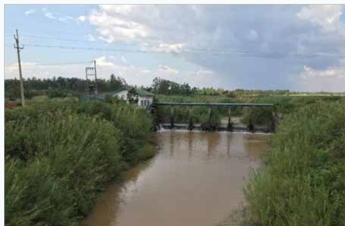
FIGURE 39: THE MUNDIKA WATER INTAKE FROM THE RIVER SIO, NEAR THE BRIDGE BETWEEN BUSIA AND BUMALA, WHICH SUPPLIES WATER TO THE PIPED WATER SYSTEM IN BUSIA.
