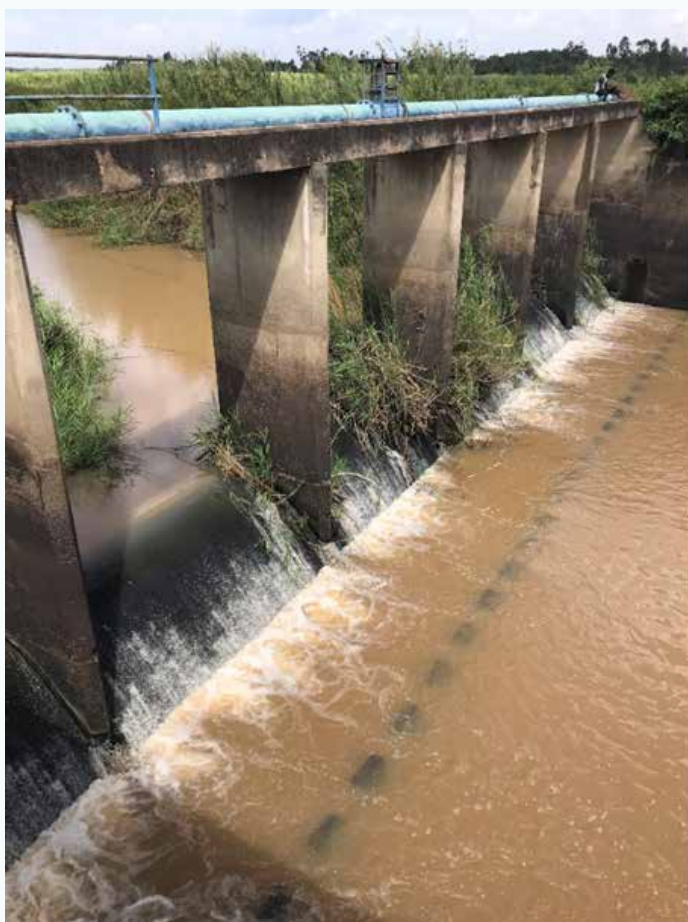
FIGURE 39: THE MUNDIKA WATER INTAKE FROM THE RIVER SIO, NEAR THE BRIDGE BETWEEN BUSIA AND BUMALA, WHICH SUPPLIES WATER TO THE PIPED WATER SYSTEM IN BUSIA.
