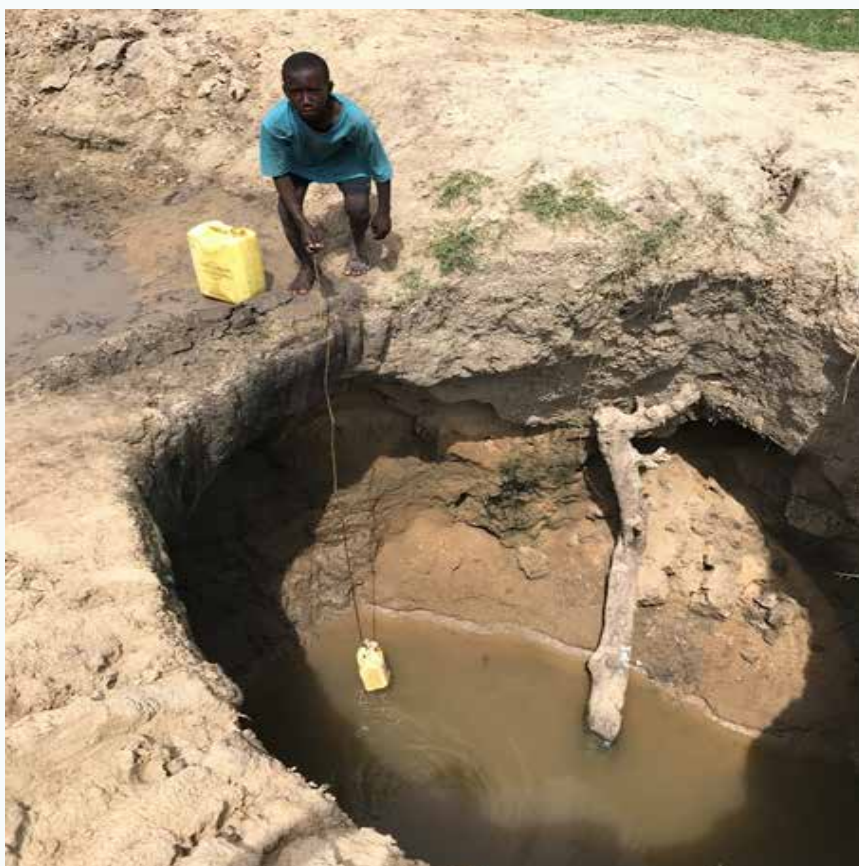
FIGURE 38: OPEN HAND-DUG WELL, USED AS SOURCE OF POTABLE WATER DUE TO LACK OF ANY PROTECTED WATER SOURCES, WITH A HIGH RISK OF FAECAL CONTAMINATION FROM THE CATTLE WATERING POINT ON THE LEFT JUST A FEW METERS AWAY. PHOTO TAKEN ON APRIL 16 TH 2019 AT LAT: 1°07'04.20" N / LON: 30°27'58.29" E.
