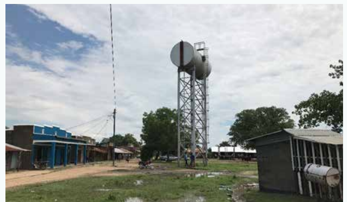
FIGURE 36: PRODUCTION BOREHOLE WITH SOLAR POWERED PUMP (PHOTO LEFT), SUPPLYING WATER TO THE ELEVATED TANK IN RWEBISENGO TOWN (RIGHT) AND FROM THERE IS DISTRIBUTED TO PRIVATE CONNECTIONS AND GOVERNMENT BUILDINGS. BOTH PHOTOS WERE TAKEN ON 15 APRIL 2019, WITH THE BOREHOLE LOCATED AT LAT: 1^{\circ}02'18.09''N / LON: 30^{\circ}15'02.66''E AND THE ELEVATED TANK LOCATED AT LAT: 1^{\circ}02'42.58''N / LON: 30^{\circ}16'20.86''E .
