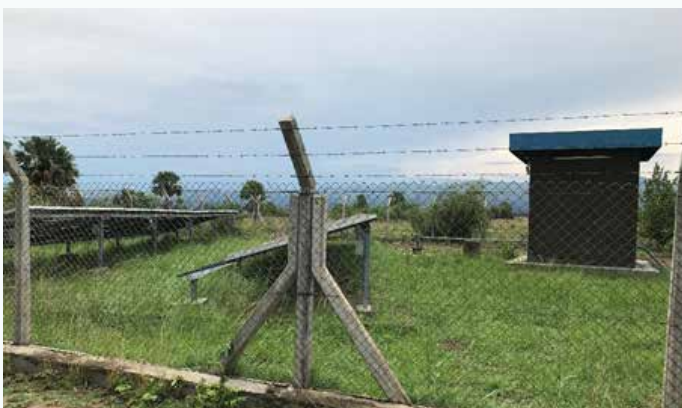
FIGURE 36: PRODUCTION BOREHOLE WITH SOLAR POWERED PUMP (PHOTO LEFT), SUPPLYING WATER TO THE ELEVATED TANK IN RWEBISENGO TOWN (RIGHT) AND FROM THERE IS DISTRIBUTED TO PRIVATE CONNECTIONS AND GOVERNMENT BUILDINGS. BOTH PHOTOS WERE TAKEN ON 15 APRIL 2019, WITH THE BOREHOLE LOCATED AT LAT: 1^{\circ}02'18.09''N / LON: 30^{\circ}15'02.66''E AND THE ELEVATED TANK LOCATED AT LAT: 1^{\circ}02'42.58''N / LON: 30^{\circ}16'20.86''E .
