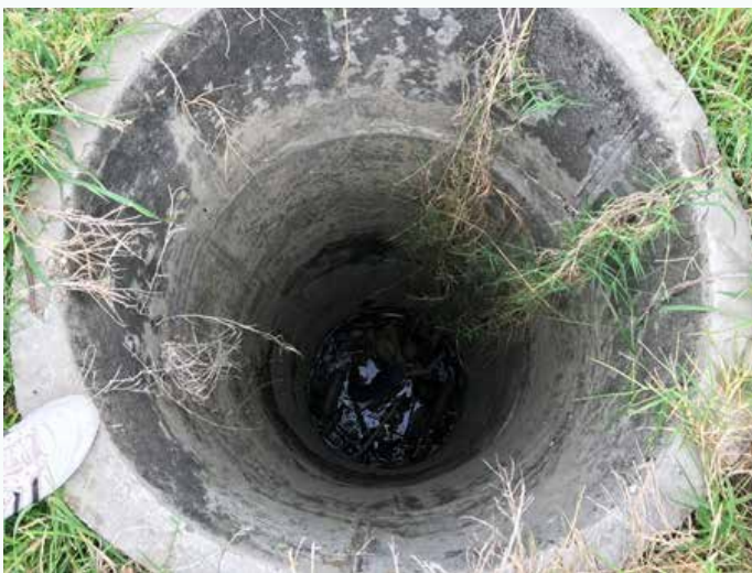
FIGURE 35: ABANDONED RING WELL FULL WITH GARBAGE (PHOTO LEFT) LOCATED NEXT TO A FUNCTIONING BOREHOLE WITH HANDPUMP, PRODUCING SLIGHTLY BRACKISH WATER ( EC = 1525\ \mu S/cm ) WITH A SLIGHTLY BROWN COLOUR (ORGANIC MATERIAL). THE WATER TABLE IN THE OPEN RING WELL WAS MEASURED AT 3,1 M BGL ON 15 APRIL 2019. LAT: 1^{\circ}05'52.31''N / LON: 30^{\circ}18'59.98''E .
