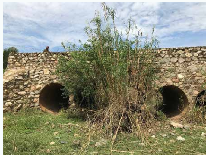
FIGURE 12: RIVER NYANJAKUFA IS A SEASONAL RIVER WHERE NO FLOW WAS OBSERVED ONLY STAGNANT WATER (PHOTO LEFT) BUT THE FIVE BIG CULVERTS UNDERNEATH THE ROAD (PHOTO RIGHT) SUGGEST HIGH FLOW WHEN THIS SIDE-BRANCH OF RIVER SEMLIKI IS ACTIVE DURING HIGH WATER LEVELS. BOTH PHOTOS TAKEN ON APRIL 15 TH 2019 AT LAT: 1°01'23.73"N / LON: 30°17'30.70"E / ALTITUDE 635 M.
