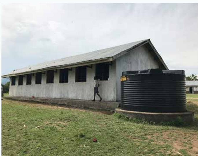
FIGURE 39: RAINWATER HARVESTING (LEFT) FROM THE ROOFS OF BUTANGAMA PRIMARY SCHOOL IS NOT FUNCTIONAL BECAUSE OF GUTS AND PIPES BEING STOLEN (RIGHT). PHOTO TAKEN ON APRIL 15 TH 2019 AT LAT: 1°04'57.54" N / LON: 30°17'35.02" E.
