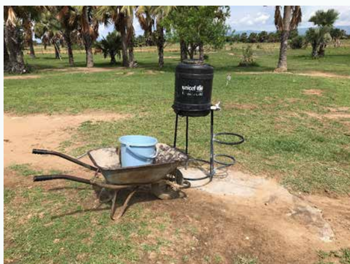
FIGURE 40: HANDWASH FACILITY AT BUTUNGAMA PRIMARY SCHOOL. PHOTO TAKEN ON APRIL 15 TH 2019 AT LAT: 1°04'58.53"N / LON: 30°17'35.23"E.
