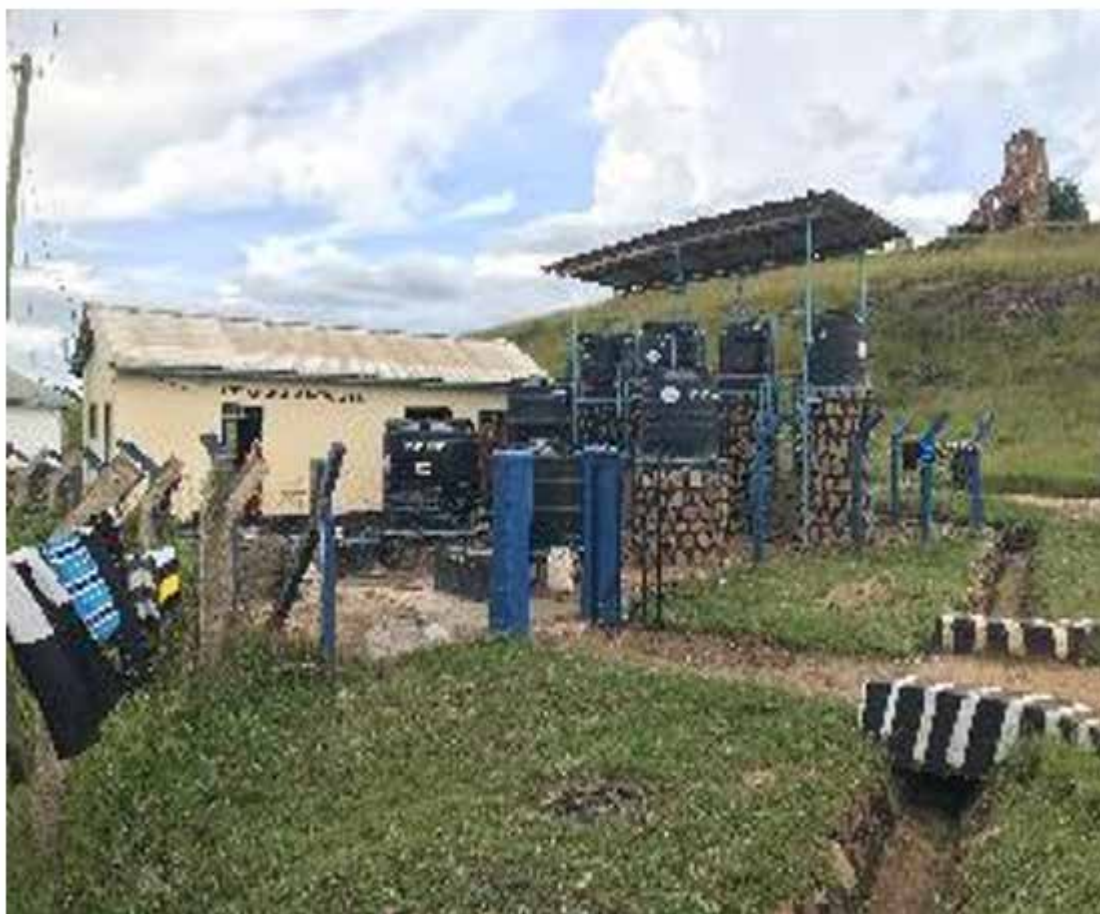
FIGURE 35: POLY-GLU DRINKING WATER KYAKA TOWN, WATER TREATMENT PLANT NEAR RIVER KAGERA. PHOTO TAKEN ON 24 APRIL 2019 AT LAT: 1°15'04.80" S / LON: 31°25'07.96" E.
