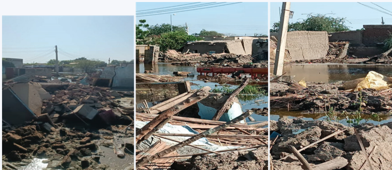
Figure 29: White Nile State flooding damages
