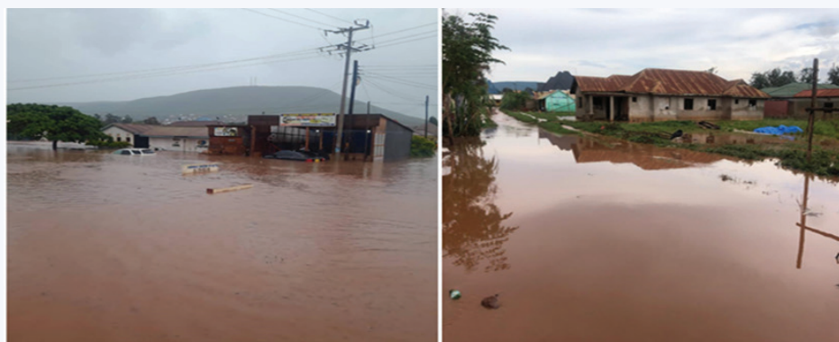
Figure 33: Flooding effect in Geita Town
