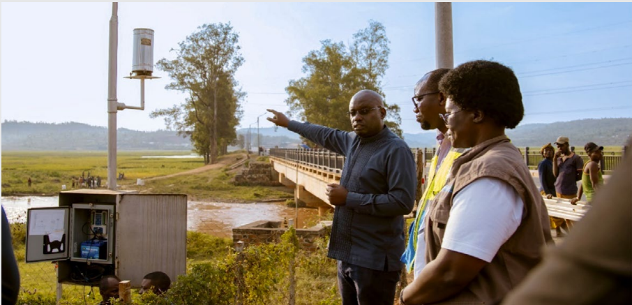
Eng. Remy Duhuze, a representative of Rwanda on the Nile TAC, explains to NBI Executive Director, Dr Florence Grace Adongo, the regional hydrological monitoring system (quality and quantity) from Gihinga monitoring station in Rwanda.
