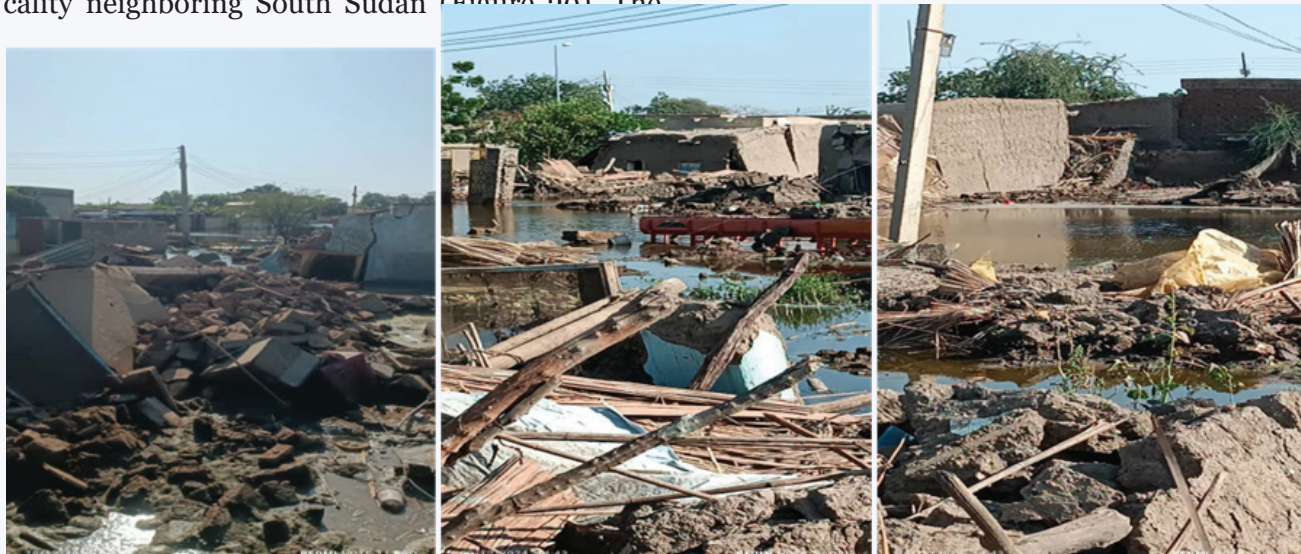
Figure 29: White Nile State flooding damages
