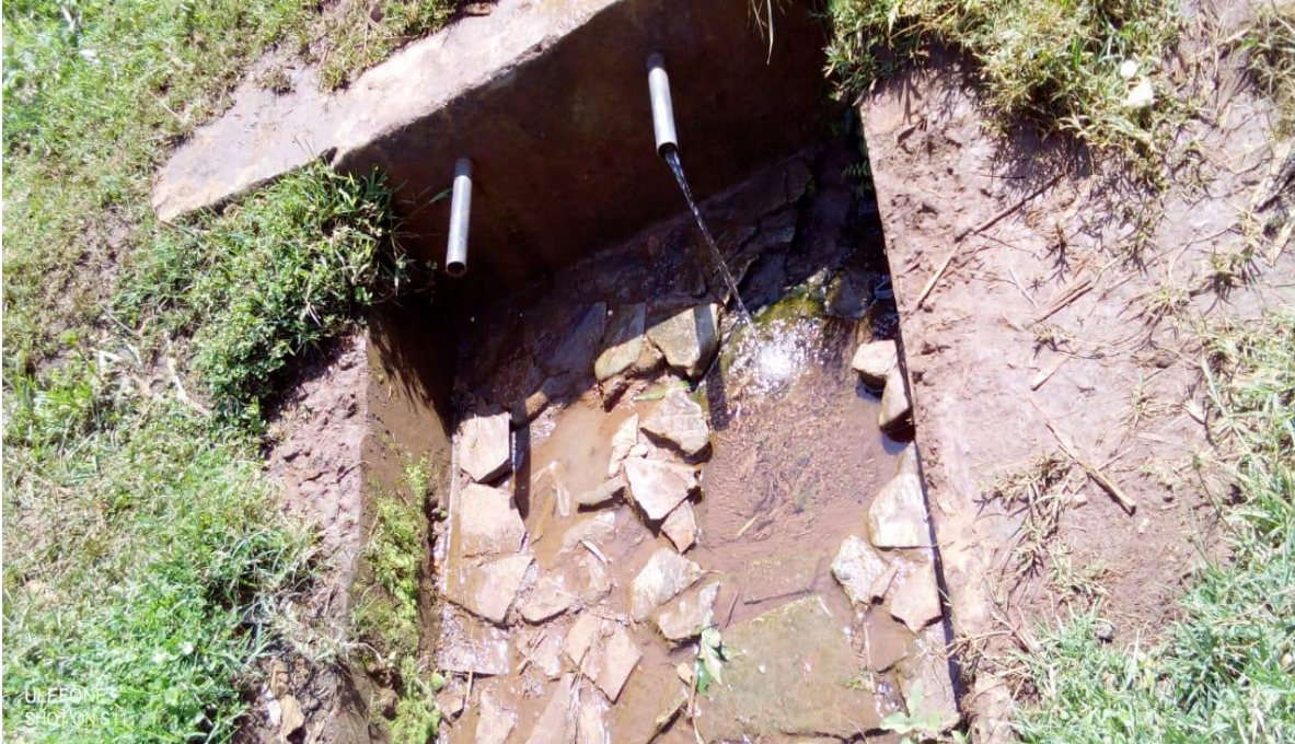
Figure 4.8: A protected spring as a natural discharge mechanism of the phreatic aquifer groundwater storage in Kenya.
