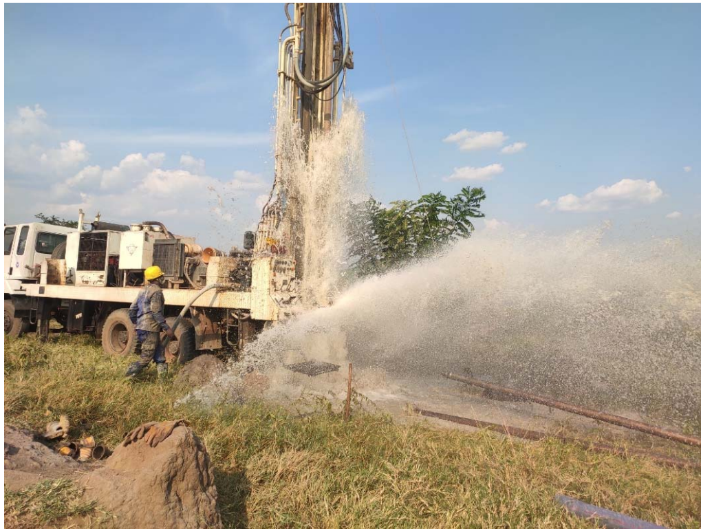
Figure 4-2: Ongoing boreholes drilling works in Ndego Sector, Kayonza (Photo)
