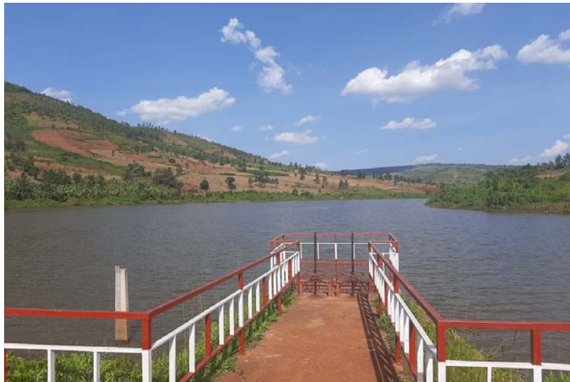
Figure 4-3: Marshland Irrigation: Sagate Dam, constructed to facilitate the farmers for the irrigation of Rice in Musaza and Gatore Sectors/ Kirehe District (Photo)
