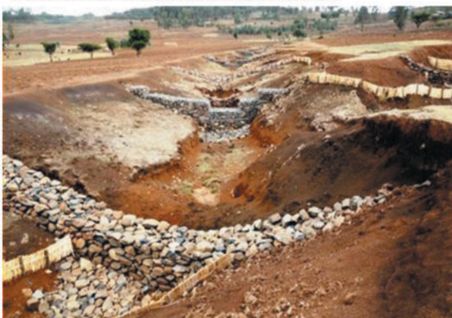
Watershed area before intervention
