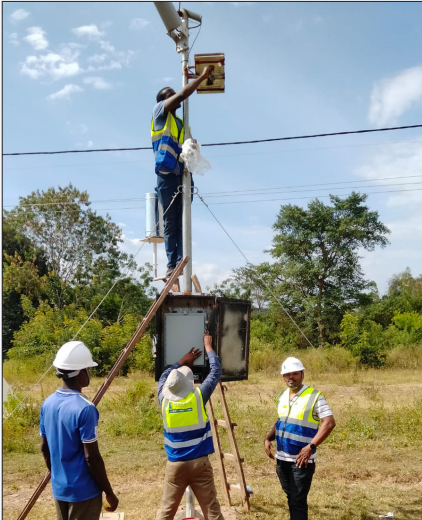
Installation of Hydromet equipment by experts in the field
