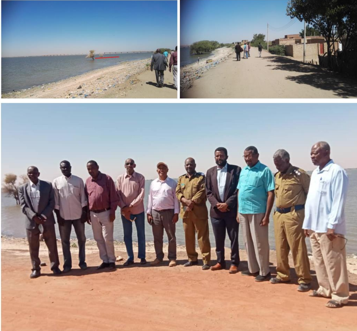
Photo: White Nile River at Jebel Aulia city - river bank (+ dyke) protecting houses (27 Jan 2023).
