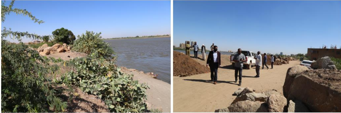
Photo: Tuti Island, 25 Jan 2023, where gully created by Nile River wave action is plugged by large stone in preparation to the July-Oct 2023 flood
