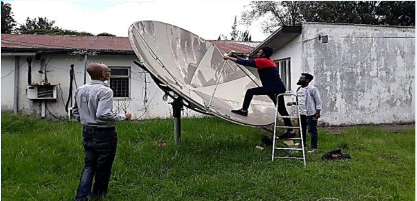
Installation of Earth Observation EO receiving dish at ENTRO.
