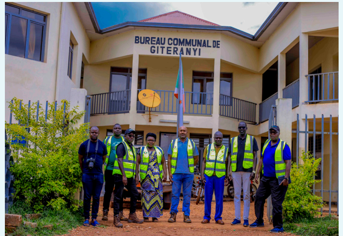
GITERANYI COMMUNE HEADQUARTERS CONSTRUCTED WITH FUNDING FROM THE LADP COMPONENT OF NELSAP RUSUMO PROJECT
