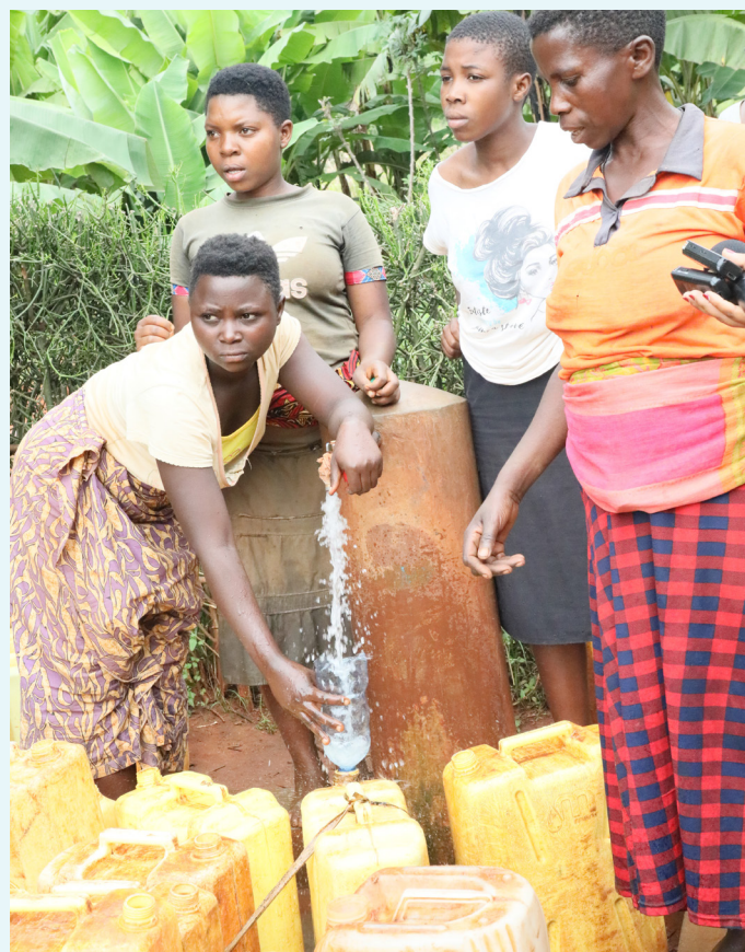
A SECTION OF REHABILITATED & EXTENDED 39 KM WATER SYSTEM IN BUSONI COMMUNE, BISHISHA, KIGERI- RUTABO
