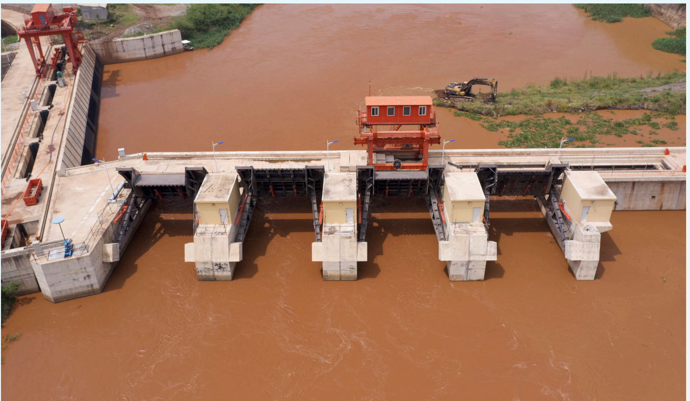
THE REGIONAL RUSUMO FALLS HYDROELECTRIC PROJECT WAS CONSTRUCTED UNDER SUPERVISION OF NELSAP-CU ON BEHALF OF THE GOVERNMENTS OF BURUNDI, RWANDA AND TANZANIA. BURUNDI WILL RECEIVE 27MW FROM THIS PROJECT
