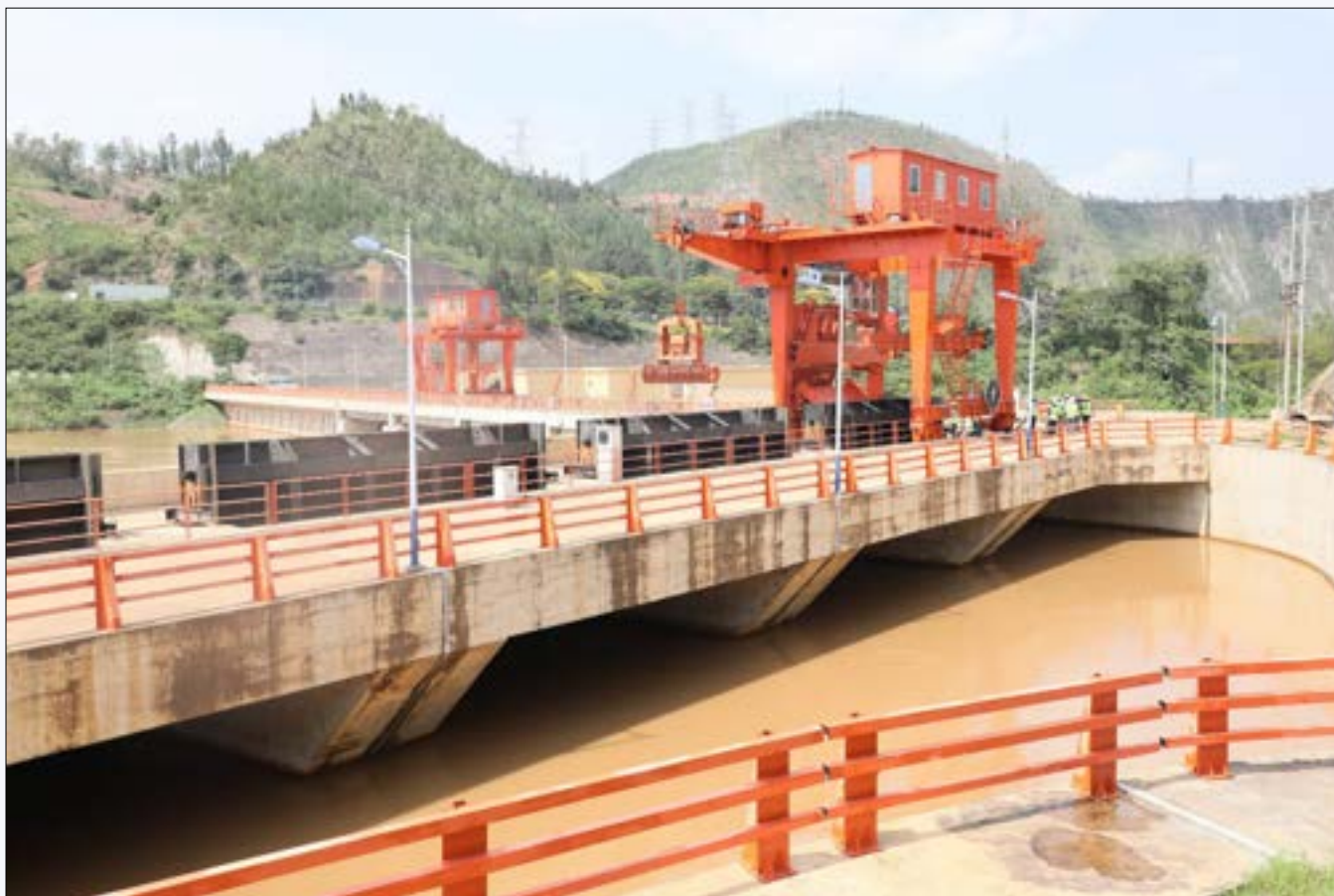
Figure 2: Radial Gates at Regional Rusumo Hydroelectric Project
