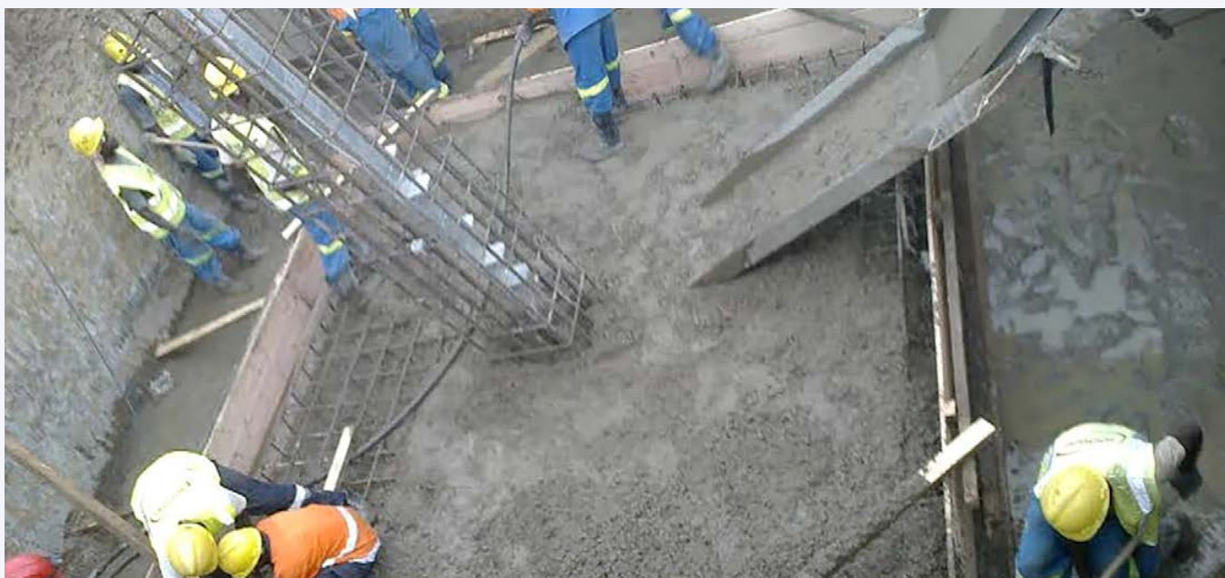
Interconnection Project. Concreting of Pad March 2015
