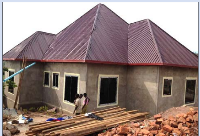
After: Arbugast Wilbard Mababu Residential house under construction
