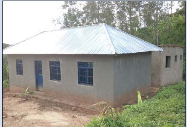
After: Residential house under finishing touches
