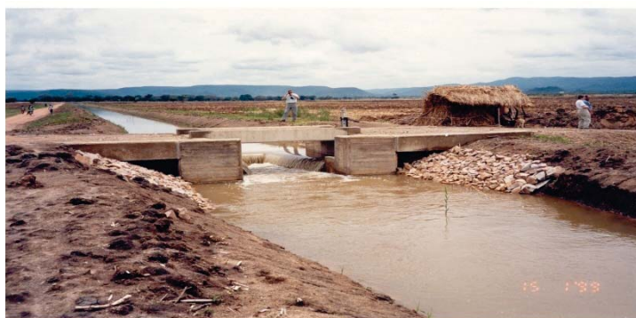
Plate 2: Canal and crossing structure at Madibira irrigation scheme
