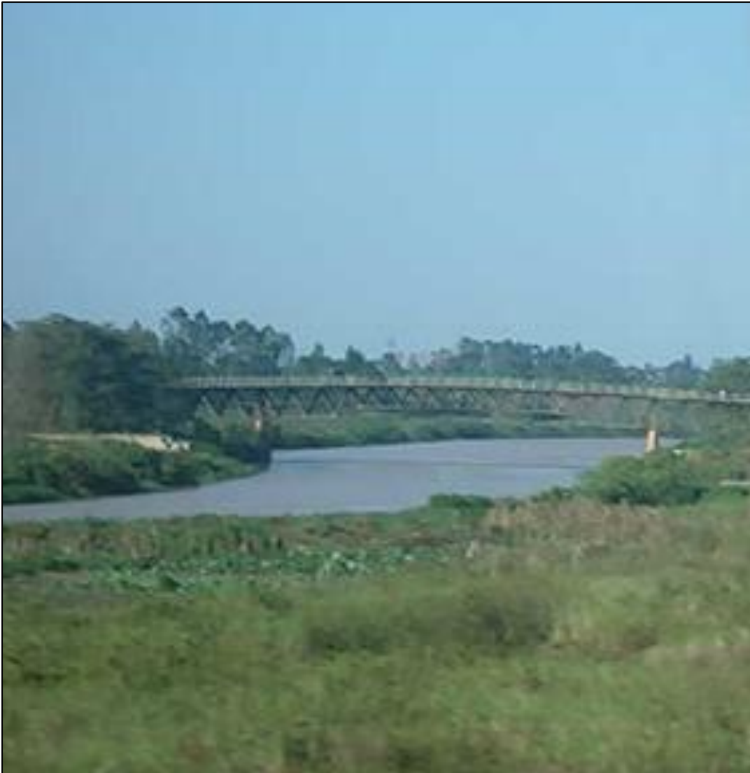
Figure 28: Photograph showing the Kagera River and associated vegetation at the bridge near Kyaka Ferry (photo courtesy of Google Earth).
