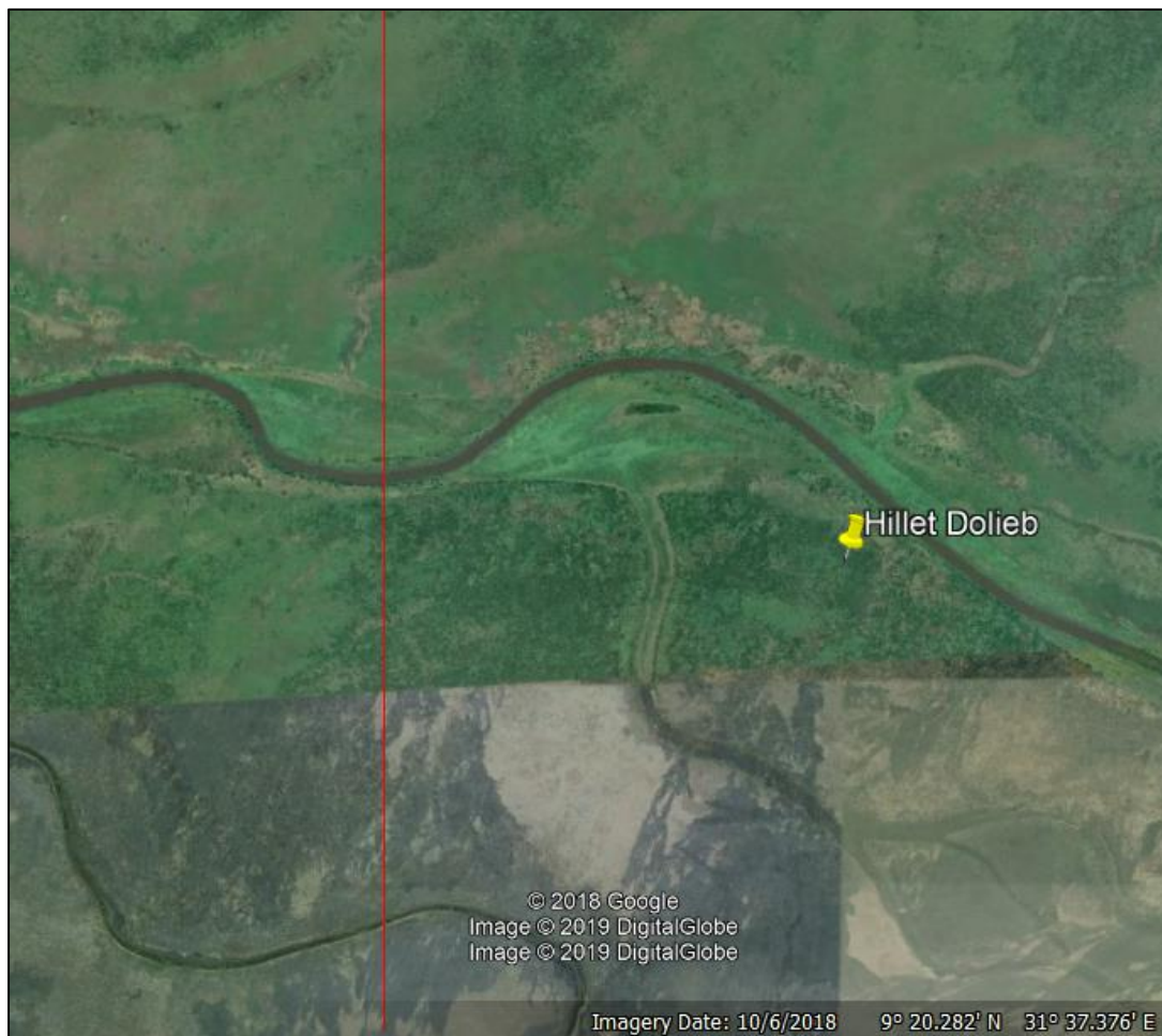
Figure 105: Google Earth © satellite image at Hillet Doleib on the Sobat River upstream of the confluence with the White Nile, representing risk region 5.
