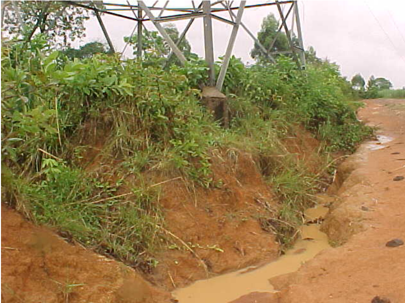
Plate: 9 Threat against the pylon foundation
