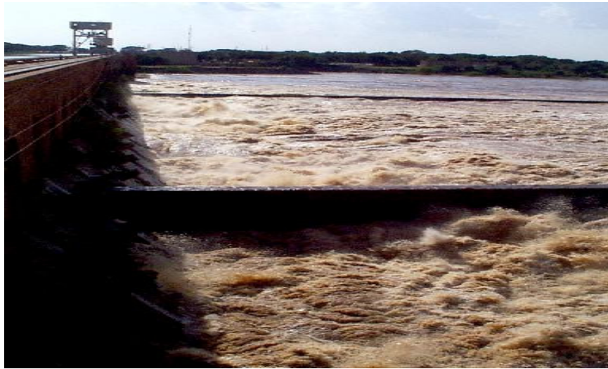
Figure 2.4: Sinnar Dam with opens gates during the flood season.
