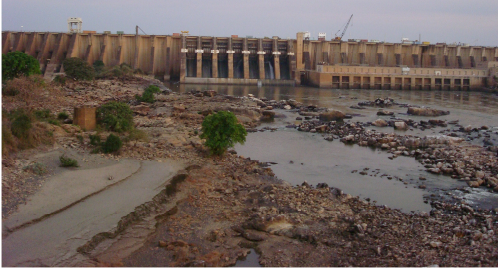
Figure 2.3: Rossieres dam with the deep sluices and spill way closed (Zaroug, 2008)
