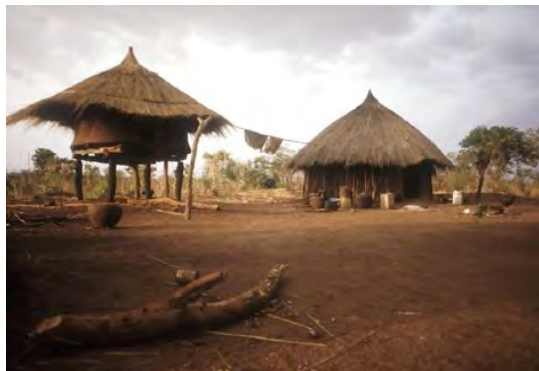
Sudan's Traditional Housing The traditional dwellings of central and southern Sudan are round, with conical roofs, and made from locally available materials. In the north, traditional houses are built from sun-baked bricks and have flat roofs.
