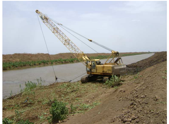
Adjacent photo shows dragline de-silting of supply canal.
