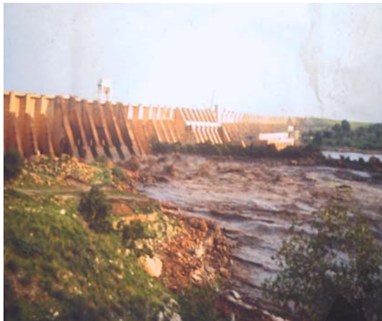
Plate(1) The Sedimentation Problem in Roseries Dam
