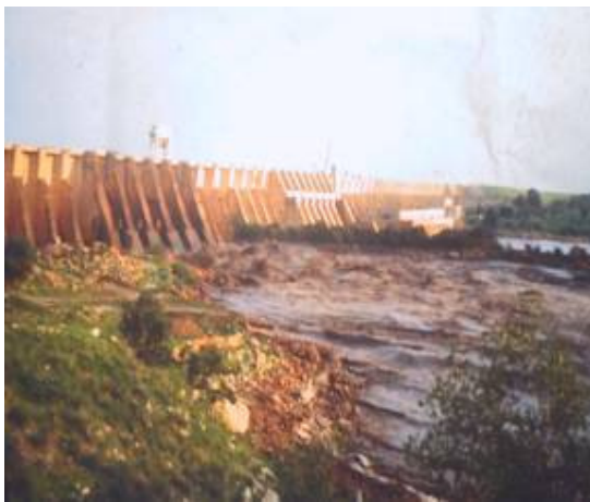
Plate (a) the Sedimentation Problem in Roseires Dam
