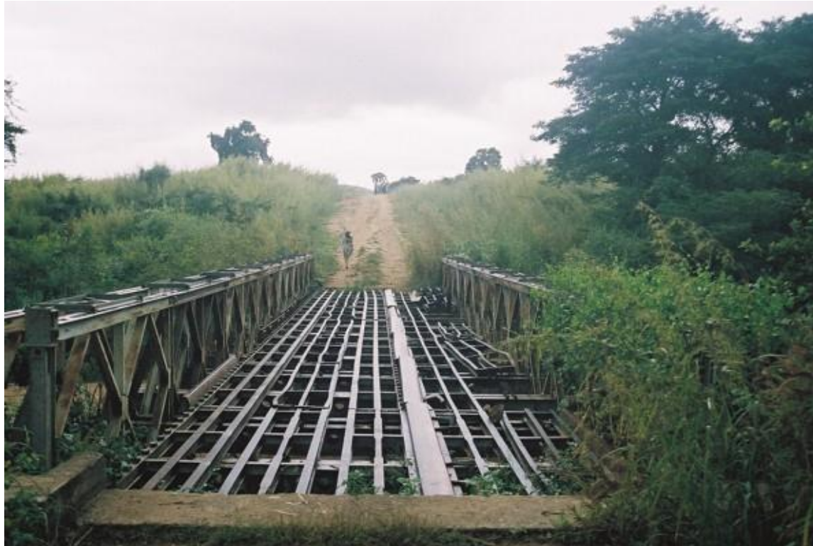
Bridge on route to Border Dam Site
