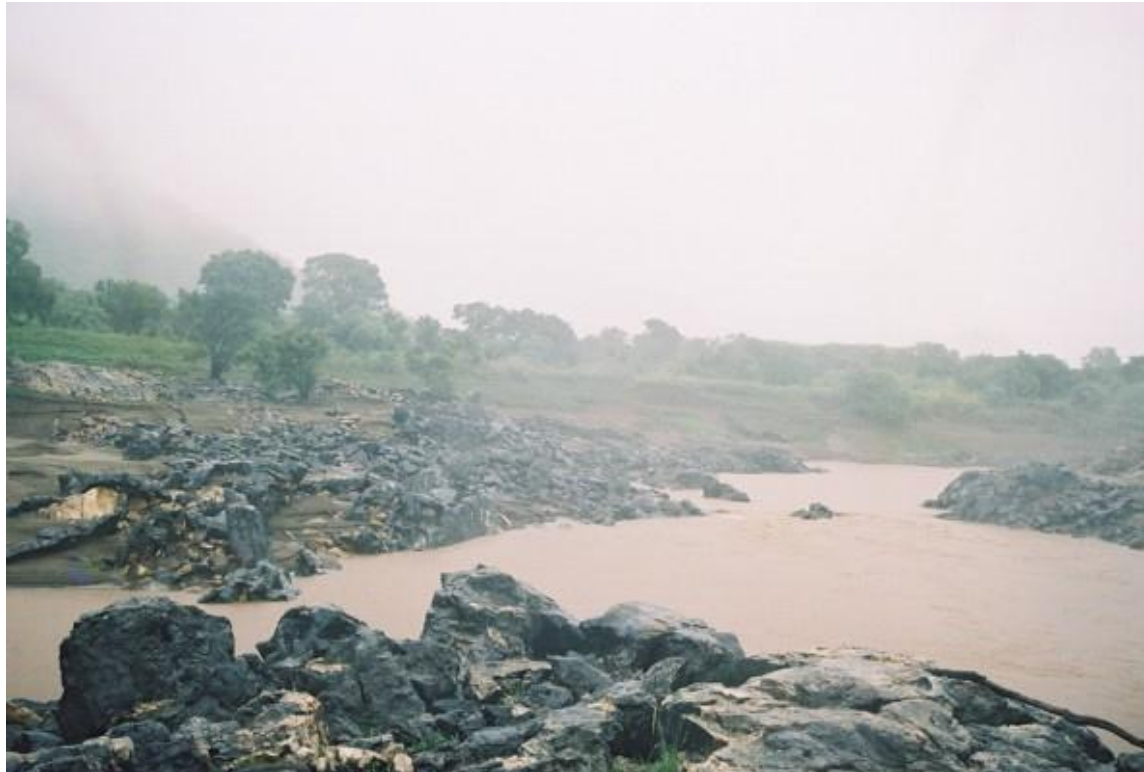
Border Dam Site – note extensive rock outcrops in river bed
