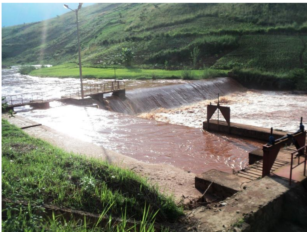
Plate 4.7-4 Diversion works from the Ruvyironza downstream of the proposed site
