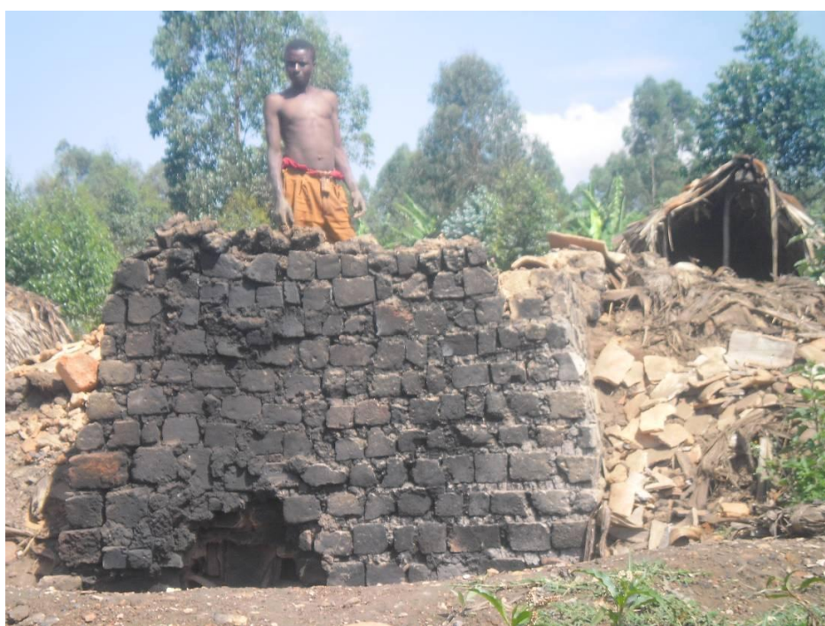
Plate 4.8-5 Brick burning near the site
