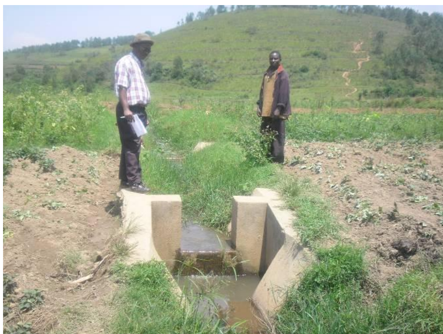
Plate 4.5-2 Part of irrigation infrastructure constructed by CRS.
