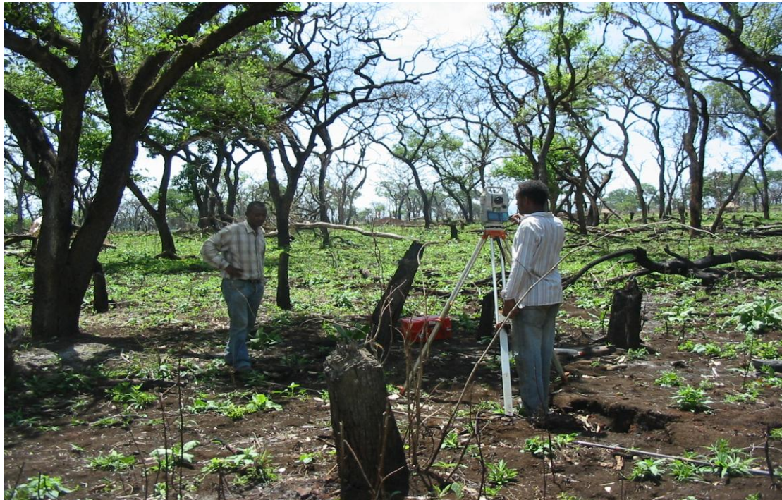
Survey of the command area in forest areas using total station equipment
