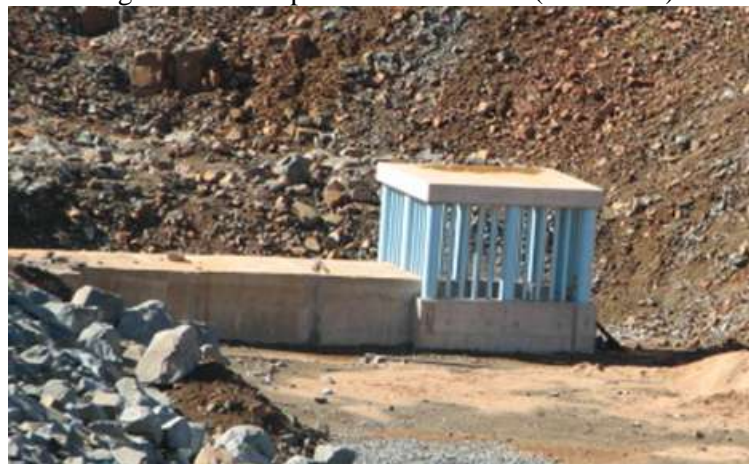
Figure 46: Example of similar intake (Swaziland)
