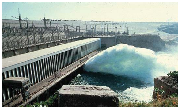
Figure 14: Lake Nasser in Egypt.
