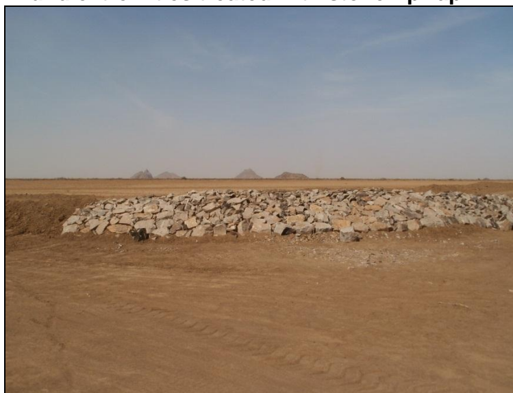
Figure 4. Bund extremities treated with stone rip-rap
