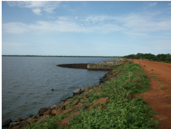
Figure 2-2: Alwero dam with security spill
