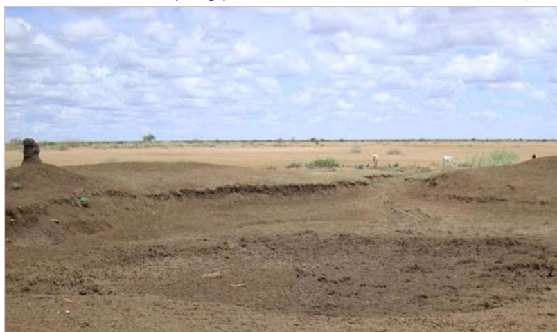
Figure 14: Siltation at community-dug ponds in the BAS sub-basin (Eastern Equatoria State)
