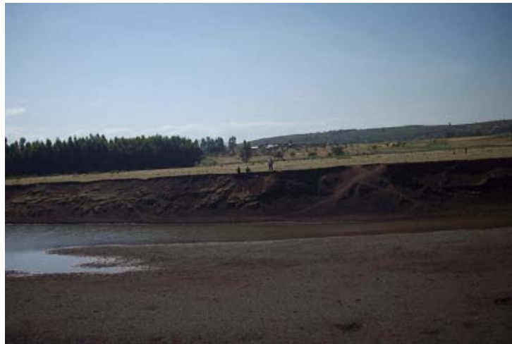
Figure 9-14: Ribb River - diversion weir area
