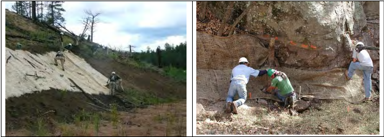
Plate 29: Jute matting to reduce soil erosion
