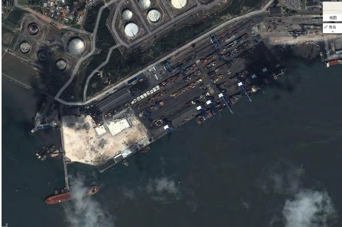
Photo 9.5.-1 Mombasa Port (Kenya)
