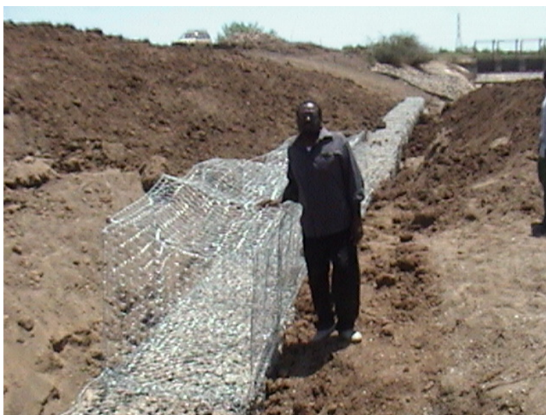
Photo 6.1: Gabions embankment in Gezira scheme
