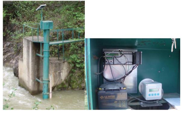
Figure 5-1: Shaft Encoder installation (left) and shaft encoder, battery and datalogger inside enclosure (right)
