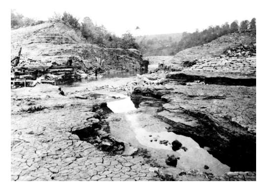
Figure 19: South Fork Dam after overtopping failure
