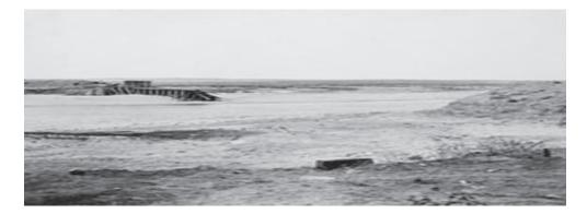
Figure 7: Avalaon Dam after its 1904 internal erosion failure
