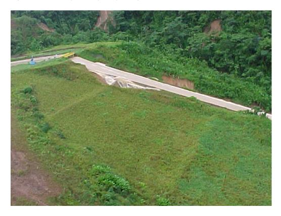
Figure 14: Overtopping Along Entire Length of Chute
