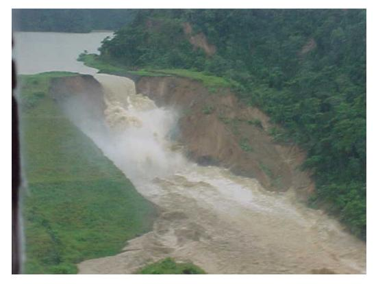
Figure 17: Breach Formation Nearing Completion
