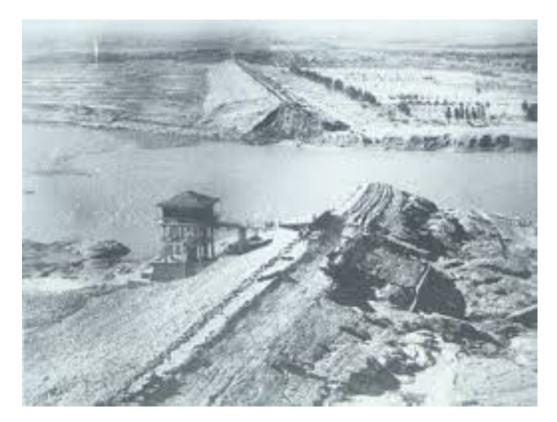
Figure 22: Banqiao Reservoir Dam after overtopping failure
