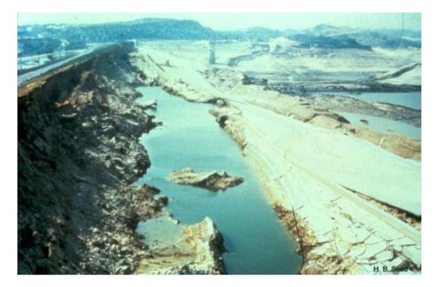
Figure 10: Lower San Fernando Dam after failure
