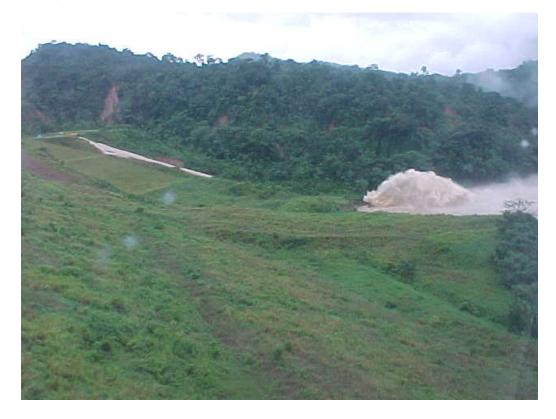
Figure 13: Sweepout of spillway stilling basin
