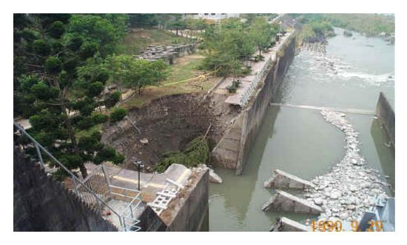
Figure 12: Failed Spillway Wall at Shih-Kang Dam
