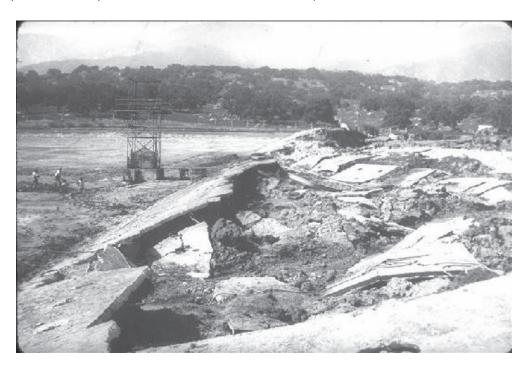
Figure 11: Sheffield Dam after seismic failure
