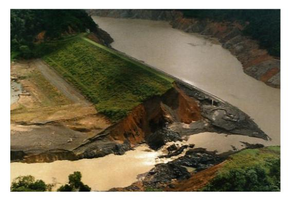
Figure 18: Aftermath of Reservoir Breach
