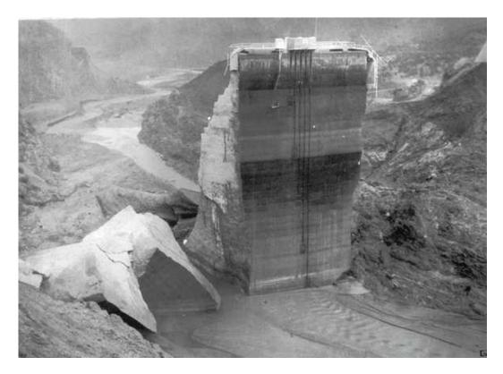
Figure 28: St Francis Dam after failure
