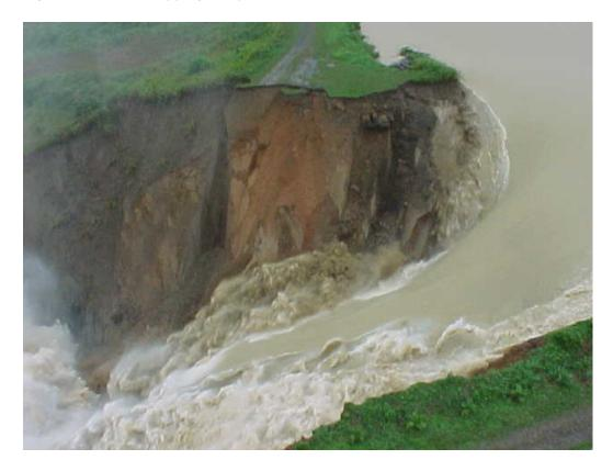
Figure 16: Headcutting Progressed to Reservoir
