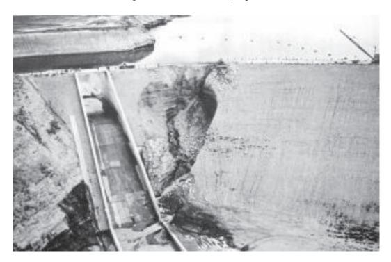
Figure 8: View of the piping at Fontenelle Dam
