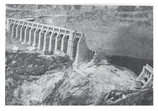
Figure 33: Gleno Dam after failure
