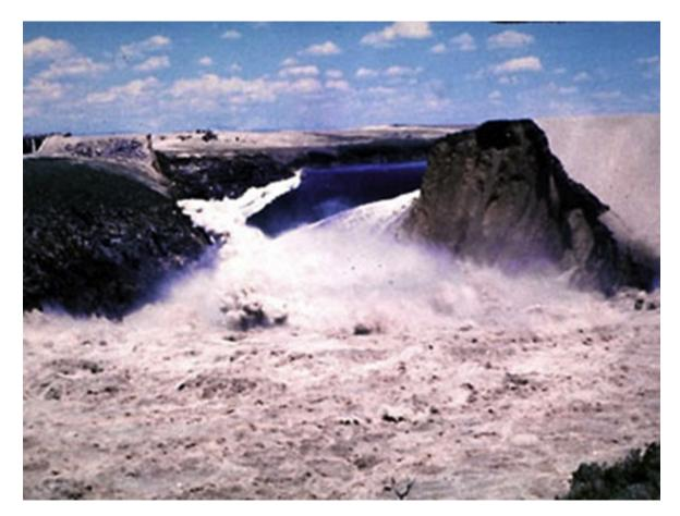
Figure 6: Teton Dam during failure
