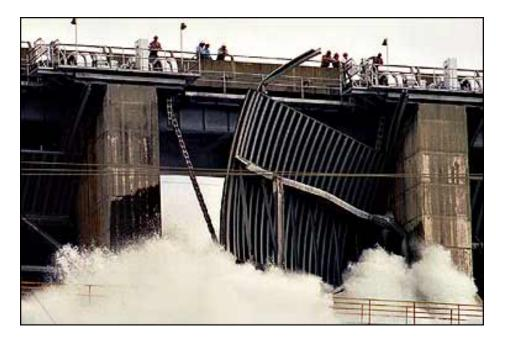
Figure 39: Folsom Dam radial gate failure
