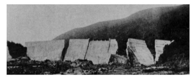
Figure 25: Austin (Bayless) Dam after failure
