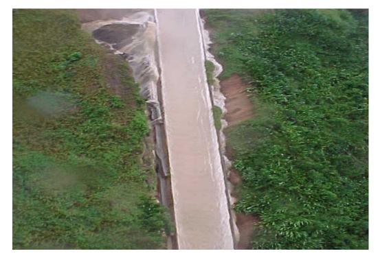
Figure 15: Overtopping of Upstream Chute Walls
