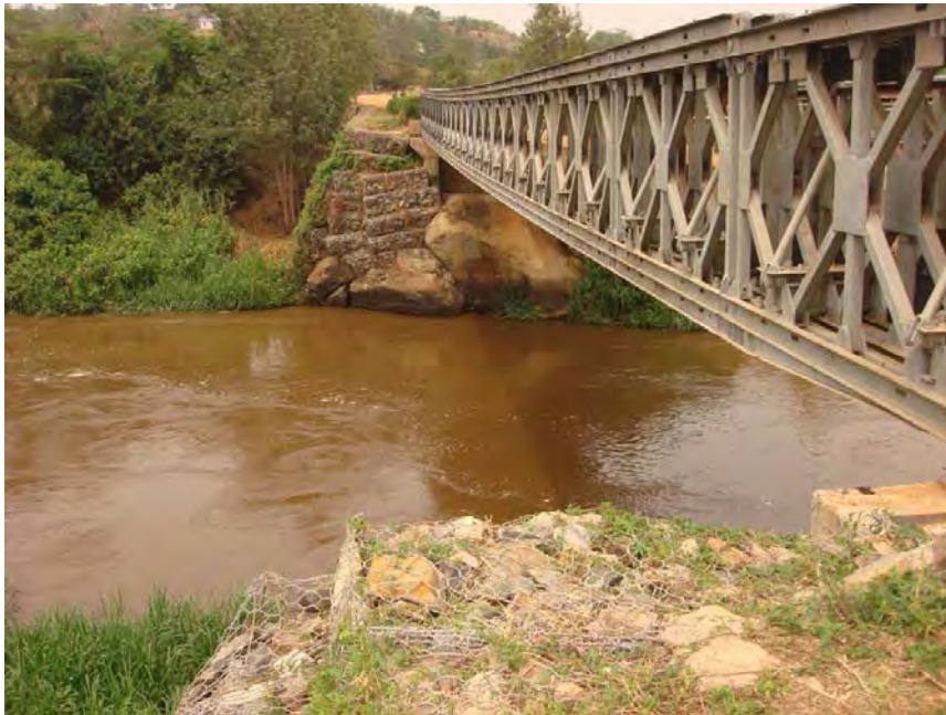
Figure 13: Bridge crossing at Murongo
